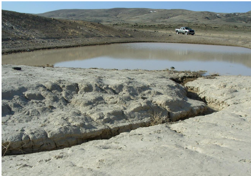
Figure 13. Severe erosion of playa surface caused by runoff into excavated reservoir. Reservoir elevation is approximately 1 m lower than playa surface elevation.
