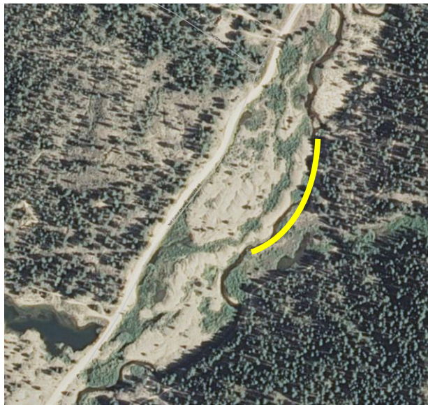
Figure 2. Restored stream reach (yellow arc), approximately 300 m long, at Grimes Creek.
