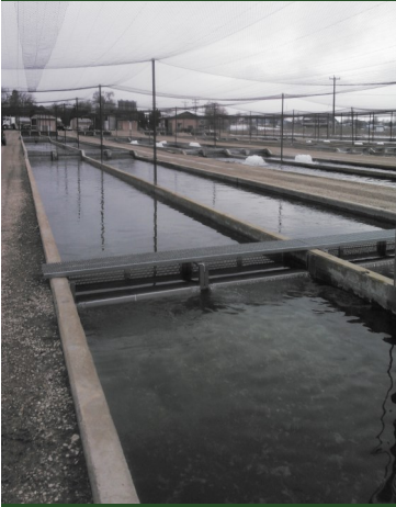
Large production raceways at Nampa Hatchery. Note: predator exclusion mesh and aeration.
