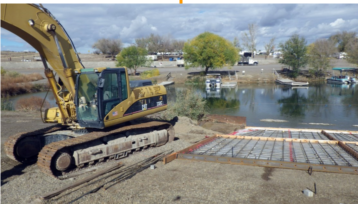
Poor-and-push technique which allows ramp blocks to be poured on dry ground and pushed into place underwater
