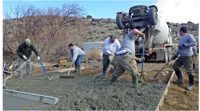
New concrete ramp being poured at Cove Arm
