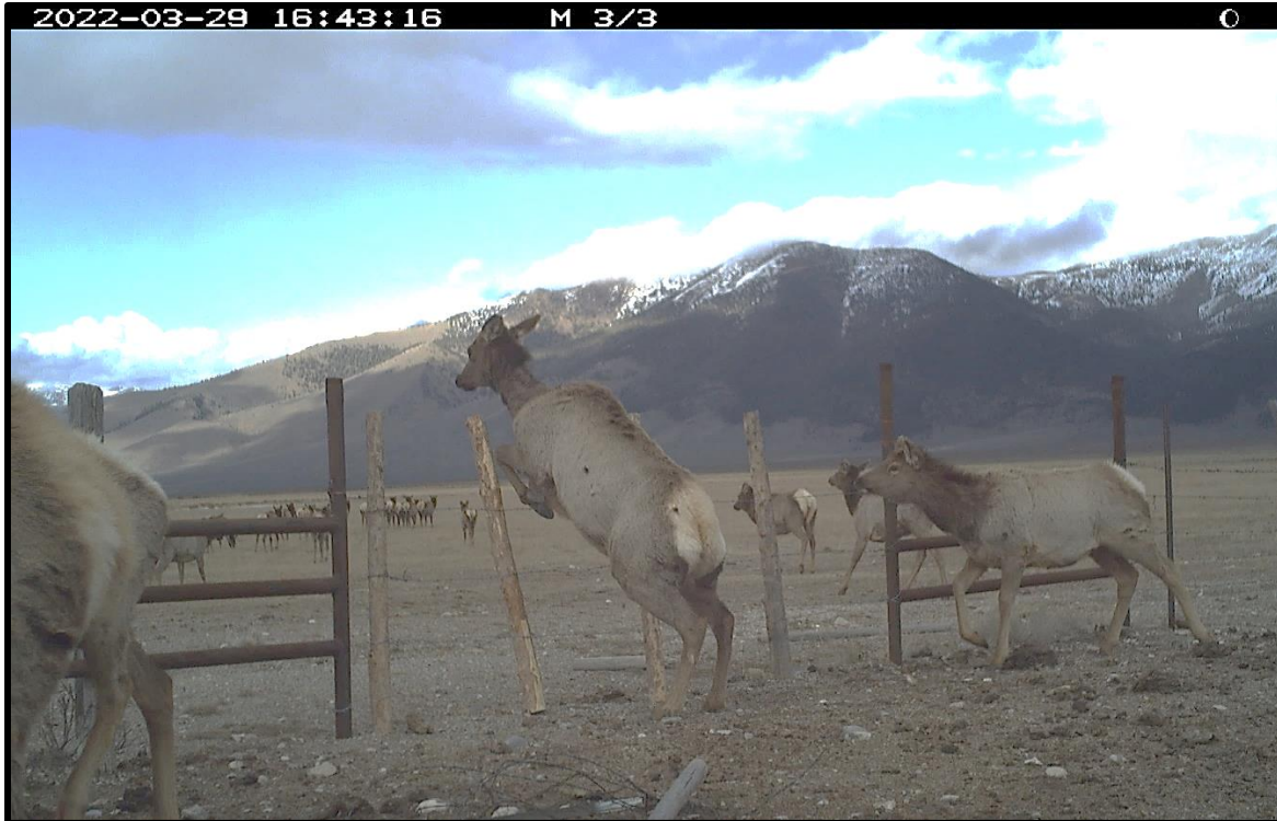
Photo 5. Wildlife friendly H-braces and gate installed in woven wire fence in the Upper Lemhi in 2021.
