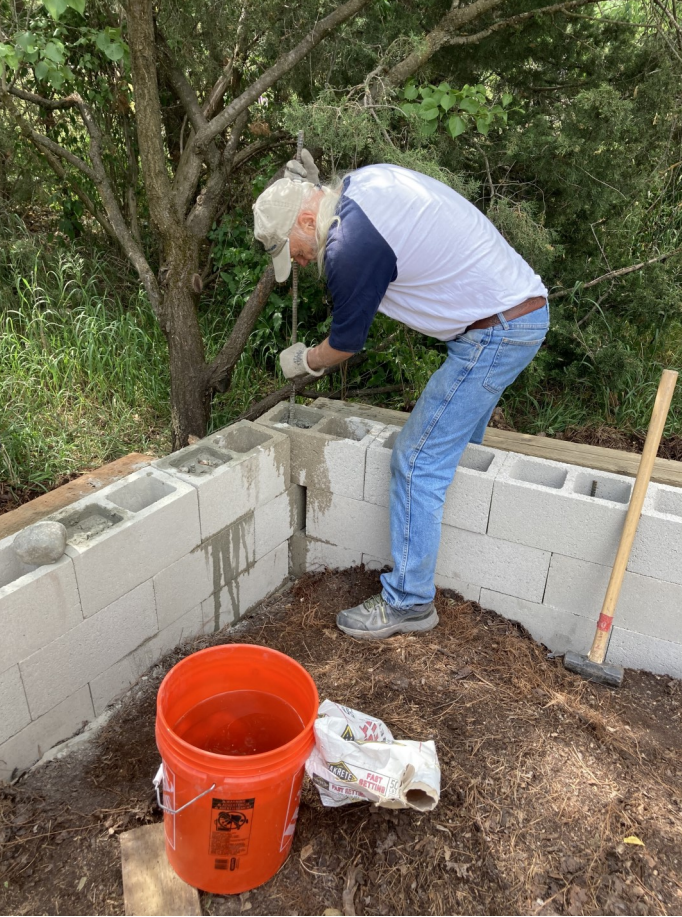
Top: Gary Hundt fortifies the walls with concrete.
