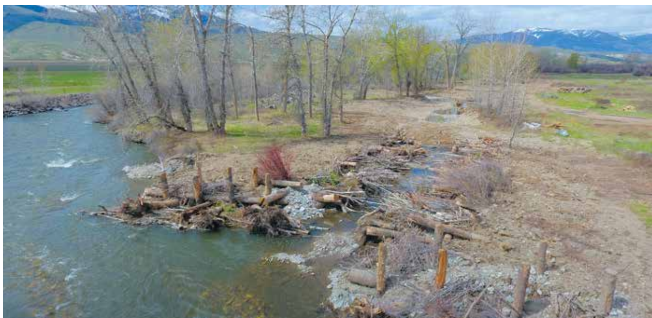
ENGINEERED LOG JAMS AND NEWLY CONNECTED SIDE CHANNELS ON THE LEMI RIVER: CC-BY IDAHO FISH AND GAME
