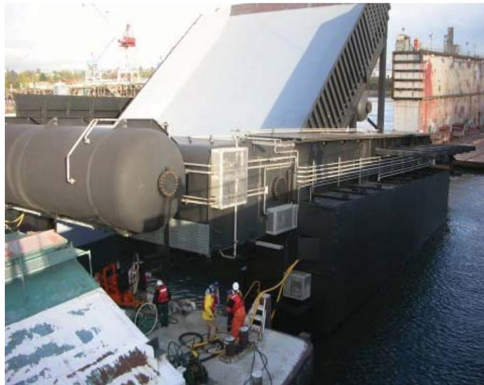
Removable Surface Weir (RSW) for Ice Harbor Dam. Photo: US Army Corps of Engineers.
